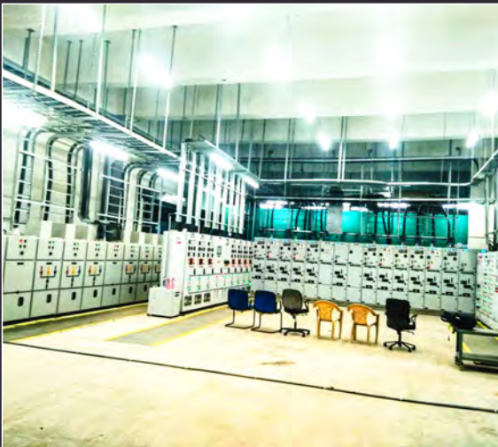
14 nos.x 2250 kVA Gensets with 11 kV Synchronized panel installed at Nextra Data centre
