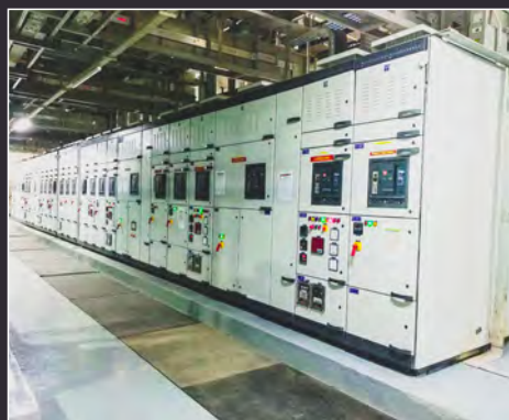
7nos. x 2000 kVA Gensets with complete Synchronization panel
