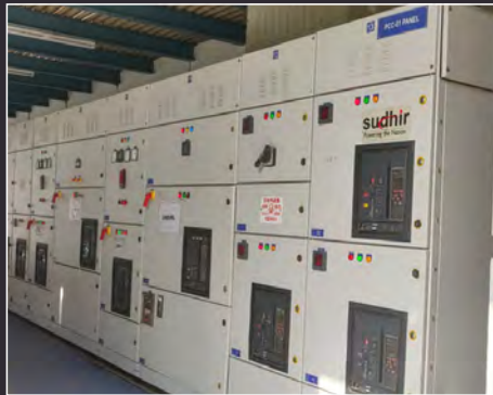
415V DG PLC based Synchronization panel, Capacitor panel, LT & Distribution panel installed at Krishna Maruti
